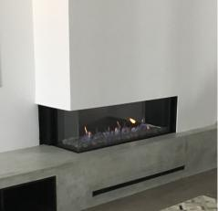
**Toe-Kick /Reveal:** A recessed opening at bottom of wall is a popular choice for air intake. It provides the option for the smallest opening. Like a gap, the opening size can be calculated to meet the square inches needed.
