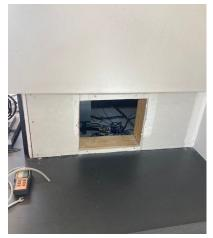
• Additionally Stone panels can be made removable for access
