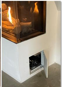
• **Hidden**: The access panel can be incorporated into the build around the fireplace. A wood panel, tile piece, or mesh screen can be made removable for servicing.
