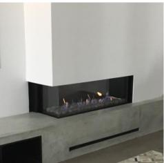
**Toe-Kick /Reveal:** A recessed opening at bottom of wall is a popular choice for air intake. It provides the option for the smallest opening. Like a gap, the opening size can be calculated to meet the square inches needed.
