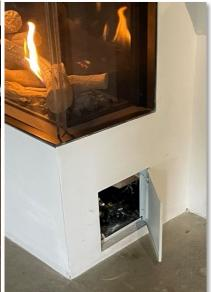
• **Hidden**: The access panel can be incorporated into the build around the fireplace. A wood panel, tile piece, or mesh screen can be made removable for servicing.
